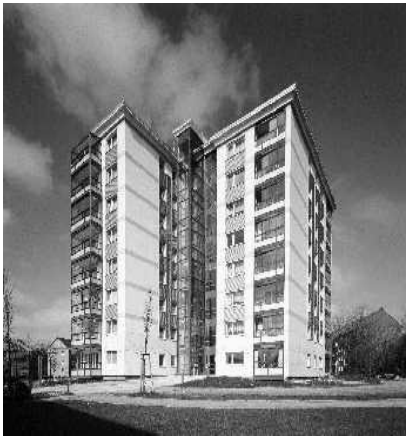
Figure 1 Refurbishment in Englesby, Germany
