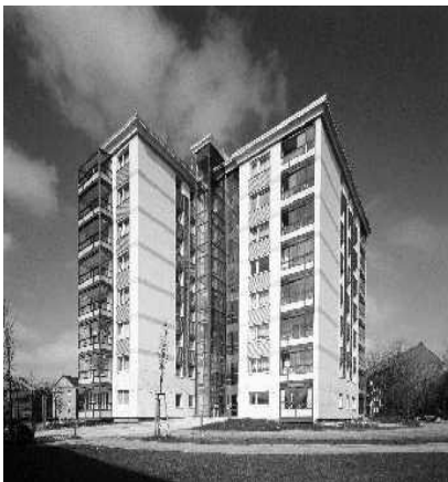
Figure 1 Refurbishment in Englesby, Germany
