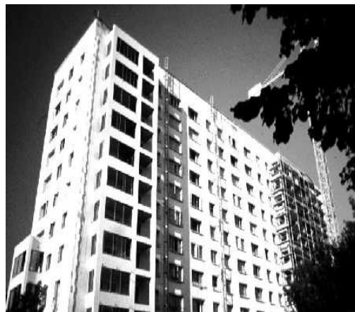
Figure 2 Refurbishment in Lyon, France
