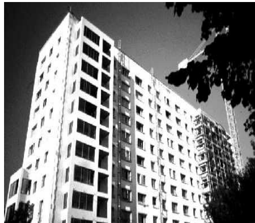
Figure 2 Refurbishment in Lyon, France
