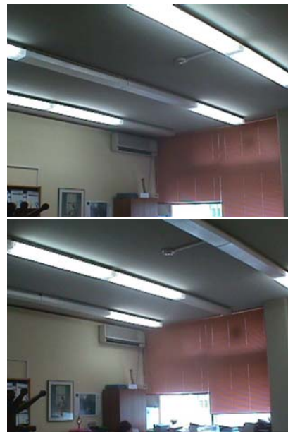
Schematic representation of the simplest switch strategy. One switch controls half of lamps.
