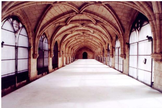
*Illustration 2: Ground floor gallery. The space is being prepared for a new exhibition. A concrete platform has been created to raise the floor by about 1.0m.*
